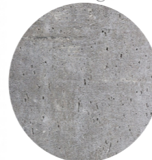
CONCRETE EXT' COLUMN
